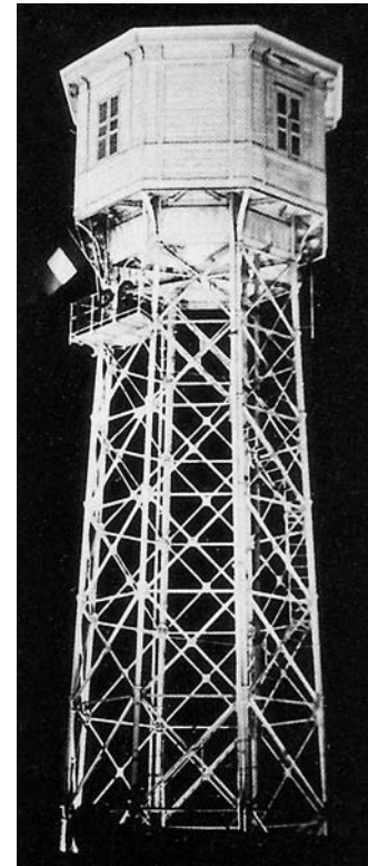
View of the imposing water cistern at the Desio silk mill complex.
