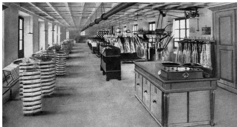
Interior view of the Gavazzi silk mill in Desio.
